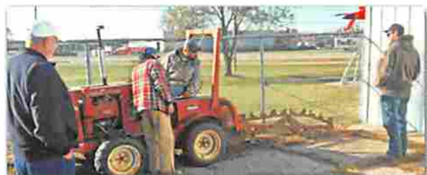
MTAA crew digging a trench between hangars 602 and 604
